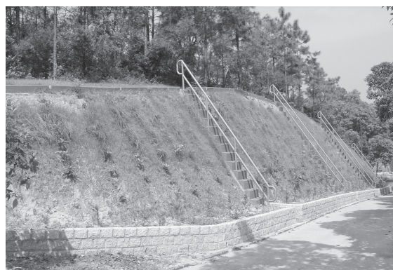
Figure 6. Part of the LPM trial site five months after hydroseeding and shrub planting
