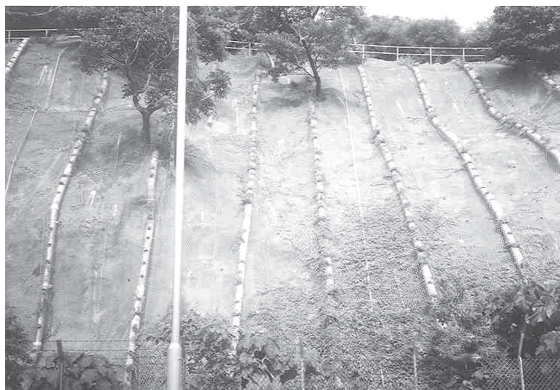
Figure 10. Hydro-planters bolted onto a steep shotcreted cut slope
